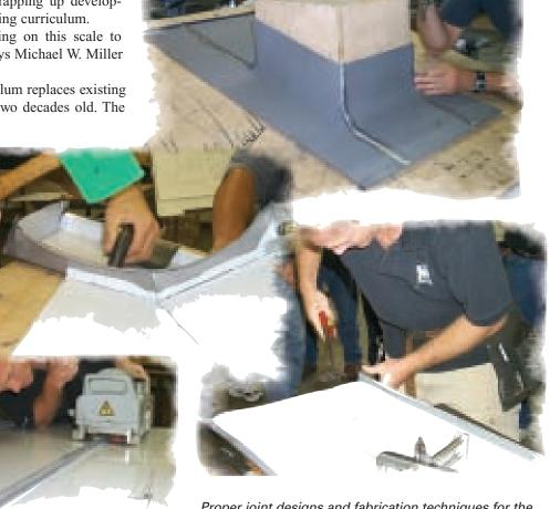
Proper joint designs and fabrication techniques for the proper installation of zinc products are covered in SMWIA-SMACNA training classes.
