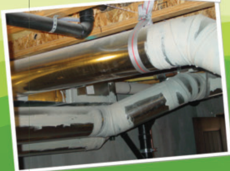
A portion of the hard duct installed in Boyer's first green residential job.
